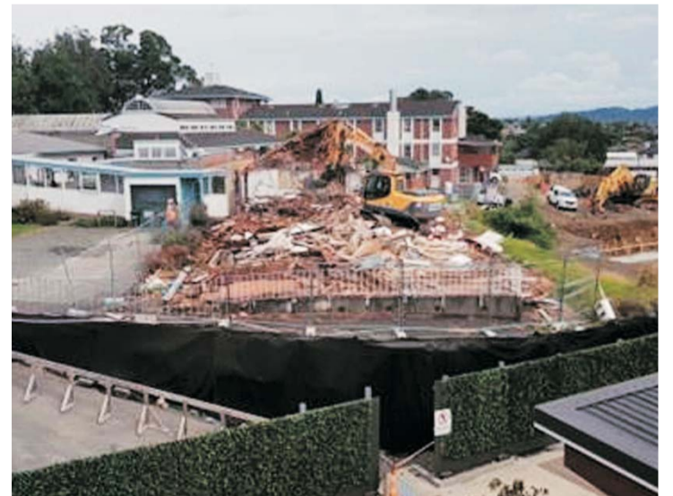
Site cleared as work begins on stage 3.
