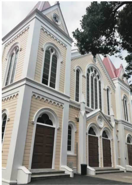
Wellington Methodist Church Seismic Strengthening almost complete.
