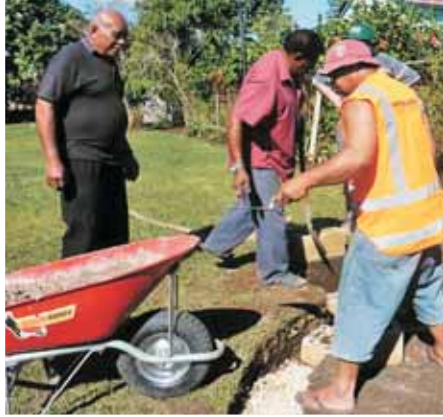
Laying down the foundations for a water tank.
