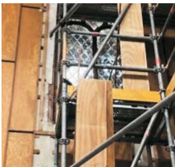
Leadlight windows will be reinstated.
