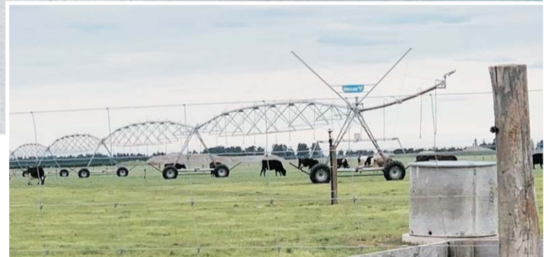
Irrigation spans. One image is only a peep into the 100's of spans and underground pipes for dairy in Canterbury. Images Betsan Martin.
