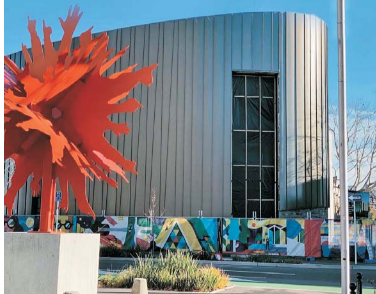
The redevelopment on the site of the former Durham Street Methodist Church, Christchurch is nearing completion.
