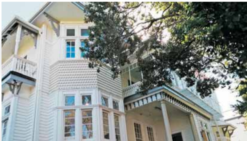
UCANZ's new home at the Anglican Centre in Thorndon.
