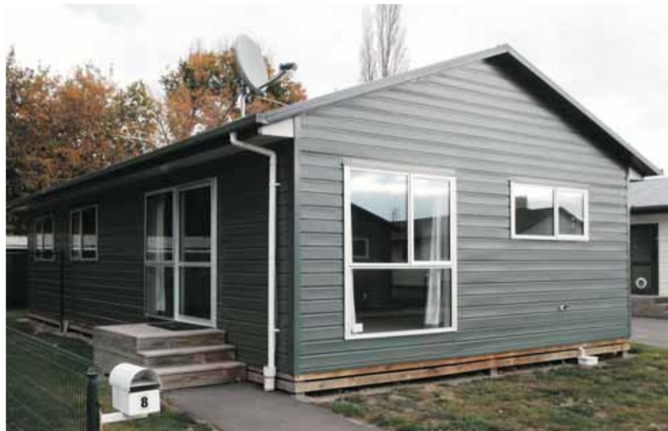
One of the relocatable houses that will provide homes to vulnerable families in Linwood.
