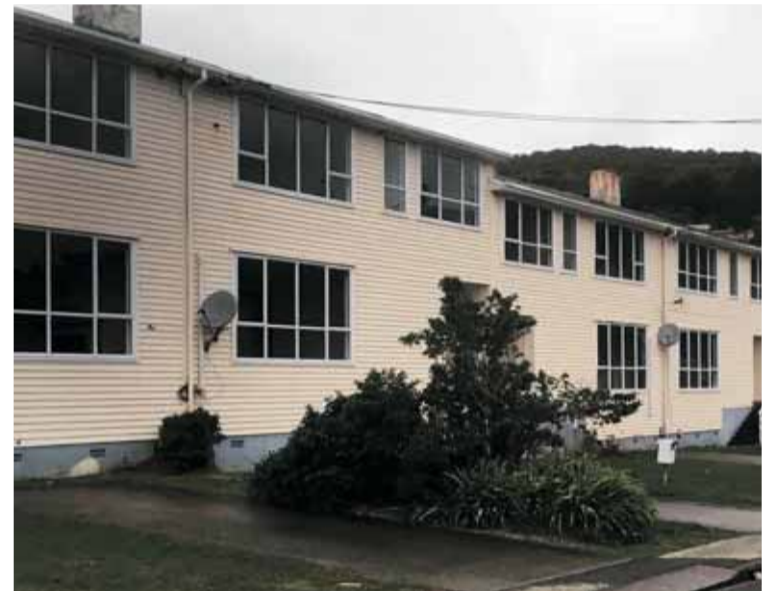
State housing in Porirua is often poorly insulated and damp.
