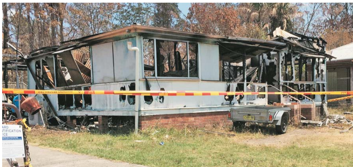
A destroyed house opposite the school. Dwellings either side of this property remained untouched by the fire path that swept through.
