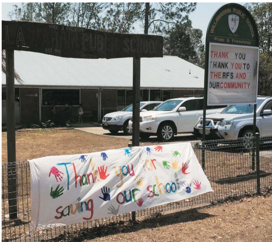
Willawarrin Public School, Willawarrin, Kempsey Shire Northern NSW. Residential properties either side of the school were destroyed.
