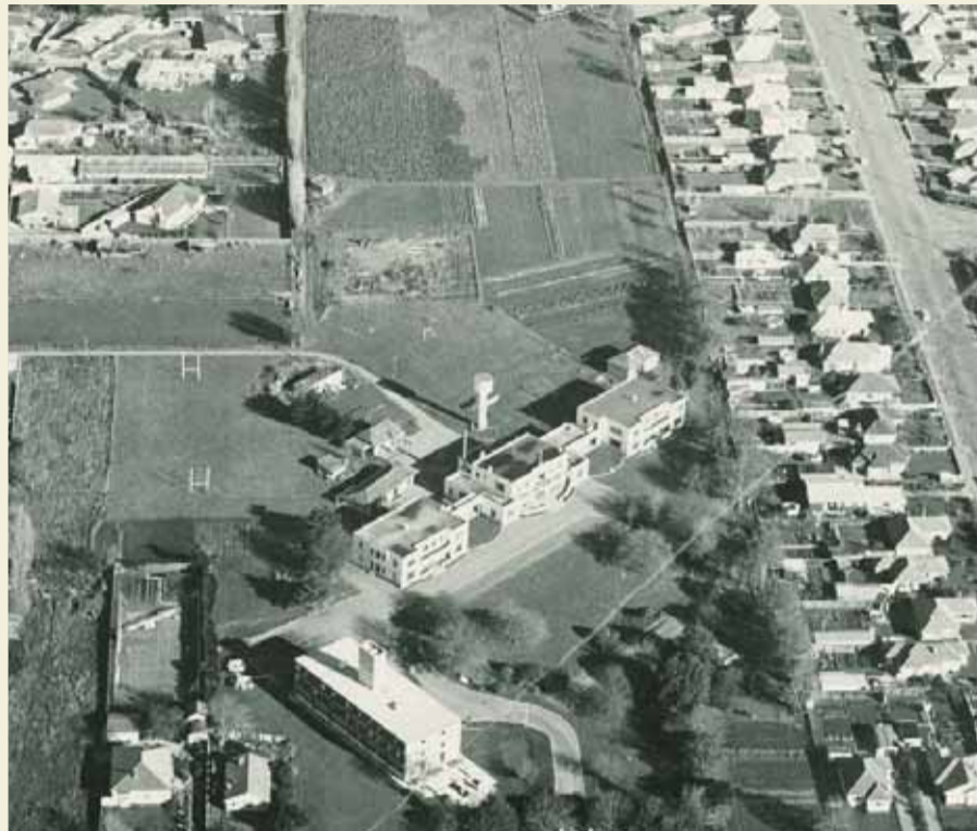
An aerial view of the South Island Children's Home in the late 1970s with the newly built Fairhaven Hospital on the grounds of the Home.
