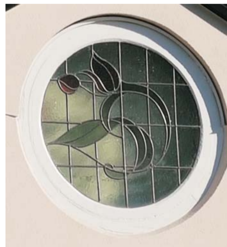
The rose window from the old parsonage is a feature of the new building.
