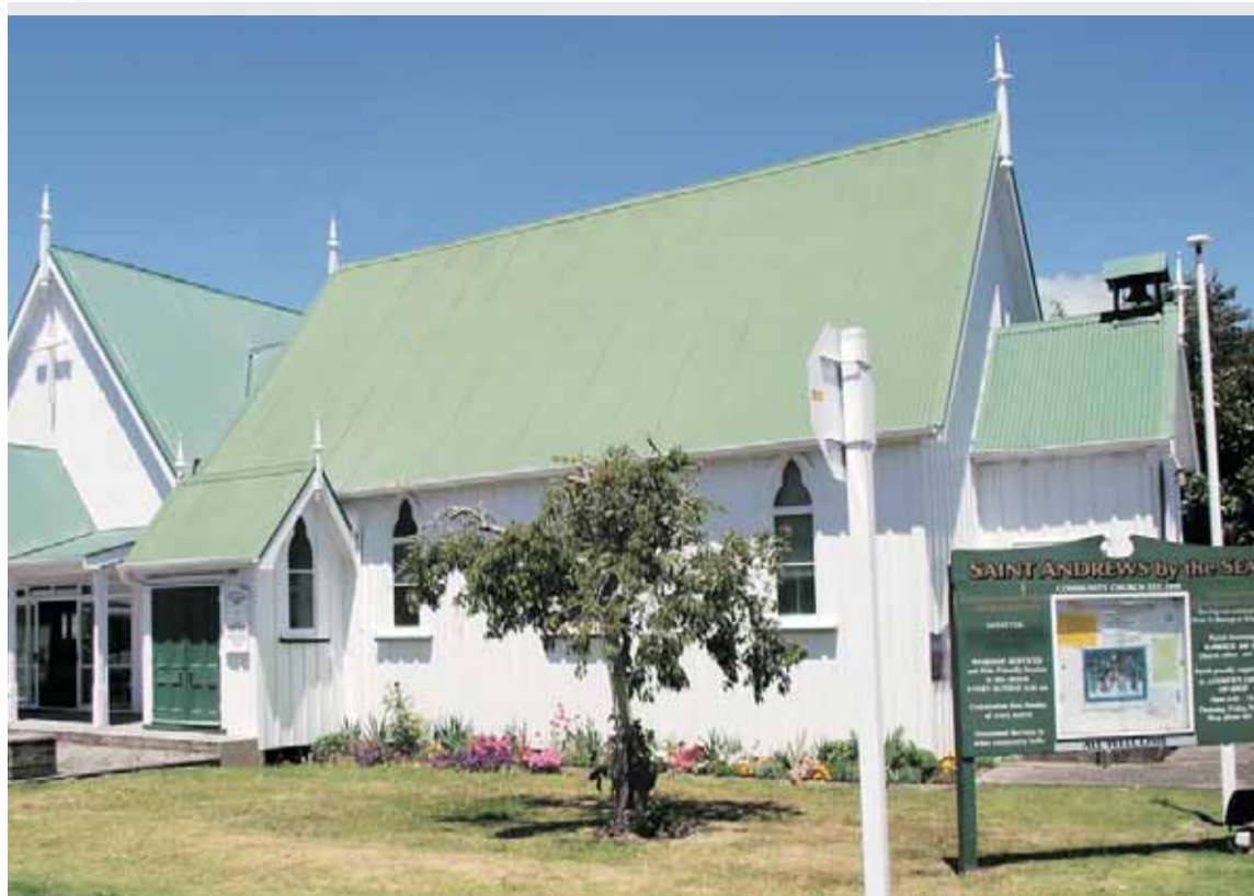
Whitianga's St Andrew's Co-operating Church has been hosting the Anglican congregation of St Peter while its buildings are being strengthened.
