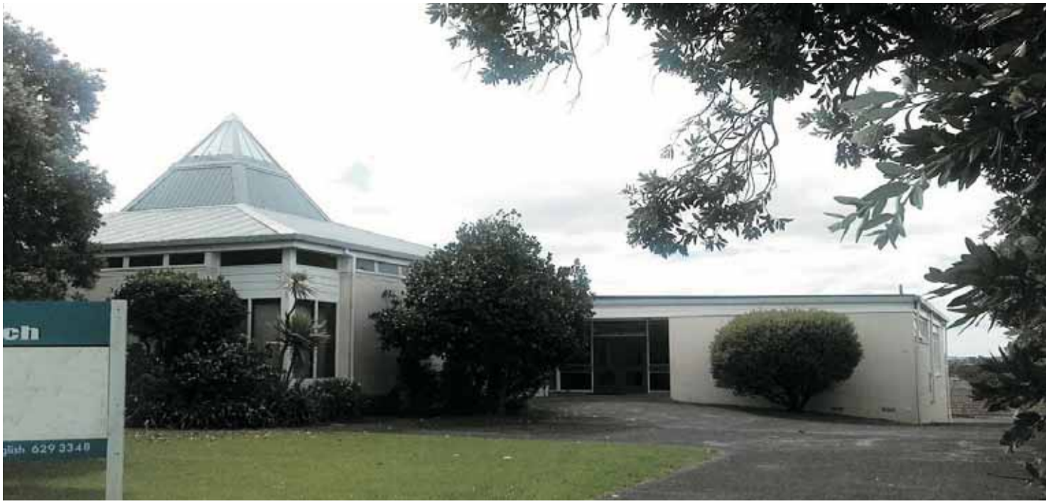
The worship space at Wesley Church Mt Roskill was unusual in its day because it was square with a central pyramidal roof rather than long and narrow.
