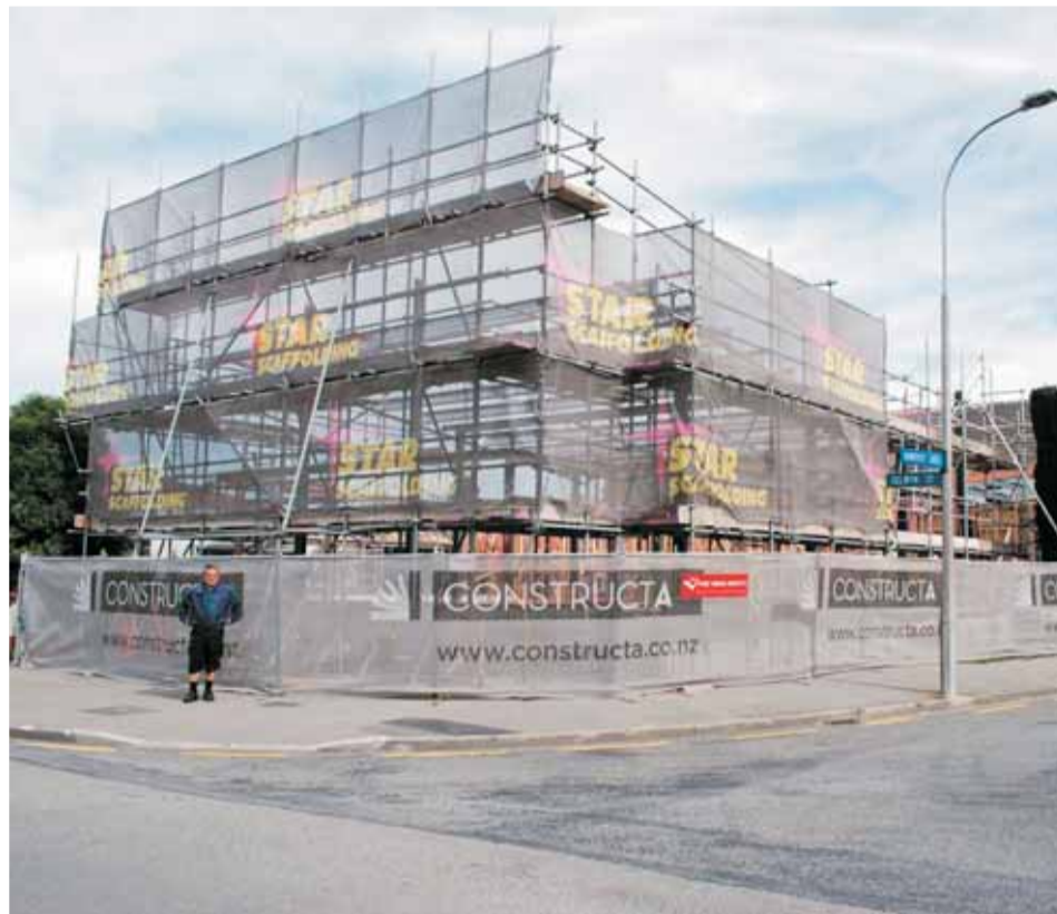
Work is underway on the Kosipeli congregation's new church hall.
