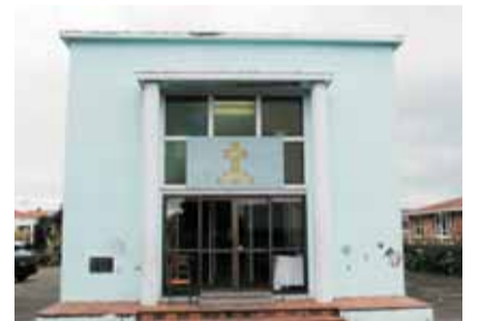
The existing church is small, cold and damp.
