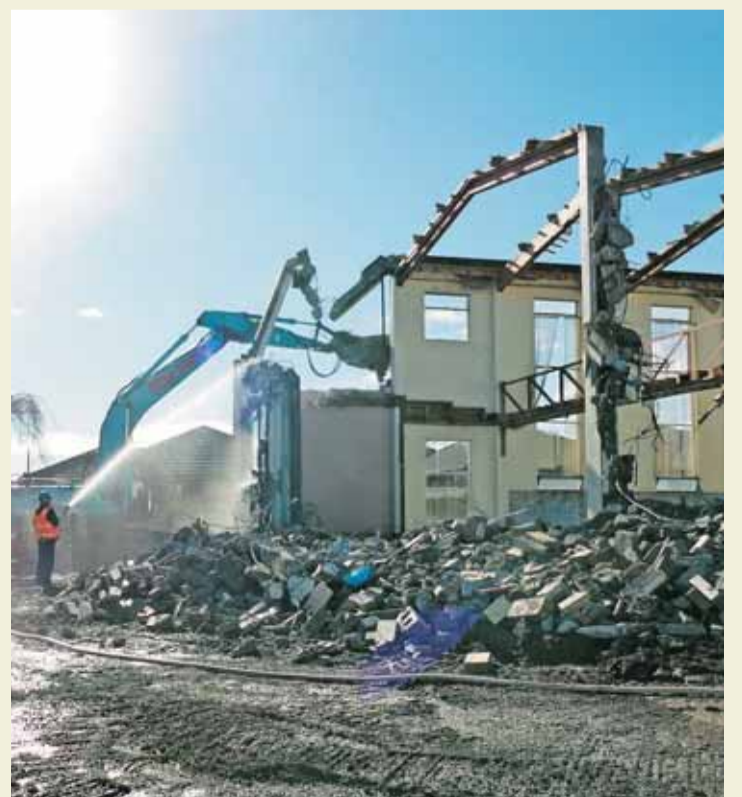
An excavator made quick work of demolishing the Stoke Methodist church.
