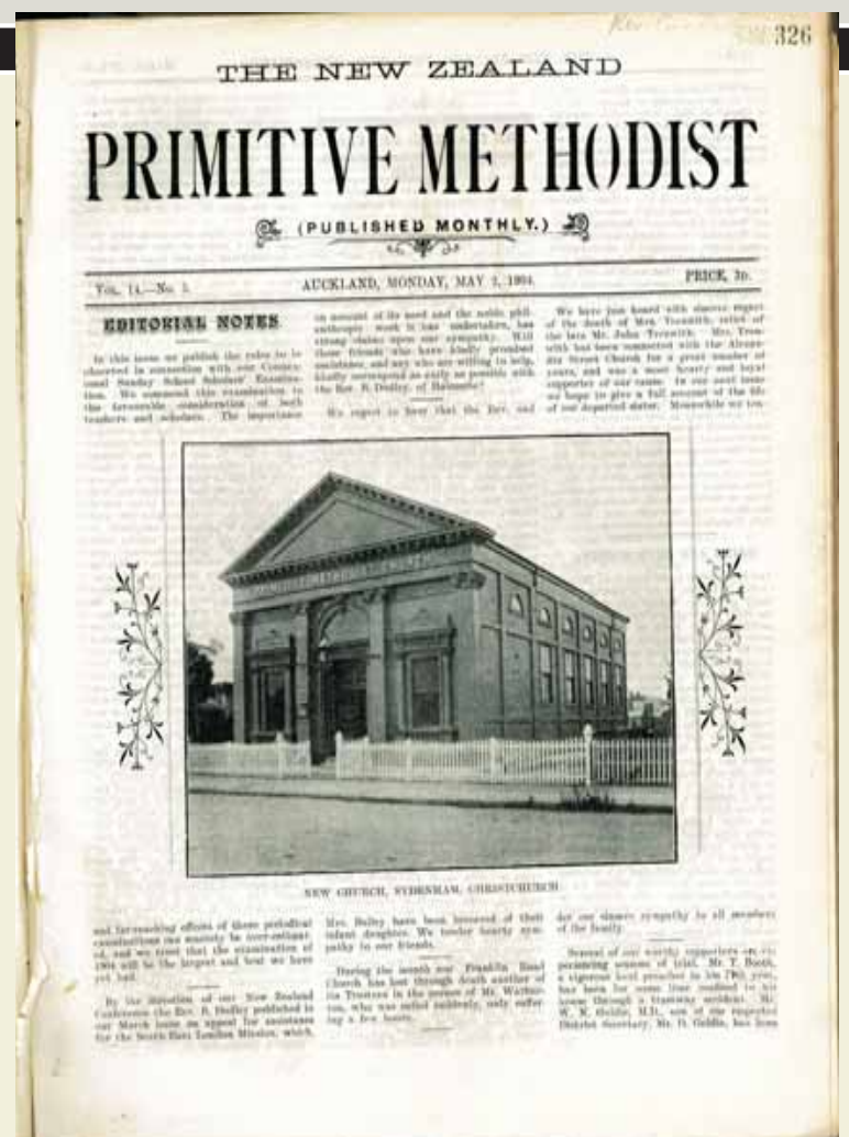
The May 1904 issue of the New Zealand Primitive Methodist celebrated the opening of the Battersea Street Church
