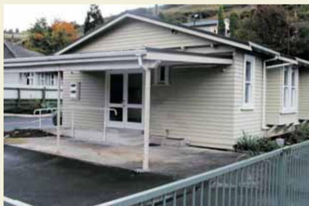
The St Lukes congregation has converted a house into a church and community centre.
