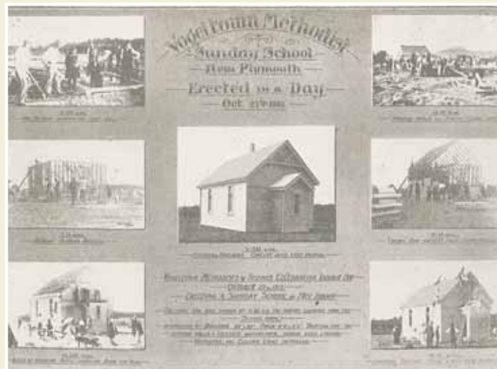
The New Zealand Methodist Times reported on the Vogeltown congregations efforts to build their Sunday school in a day.
