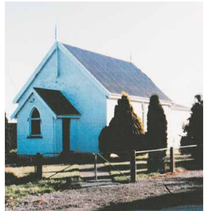
Winchmore District Church, Ashburton.
