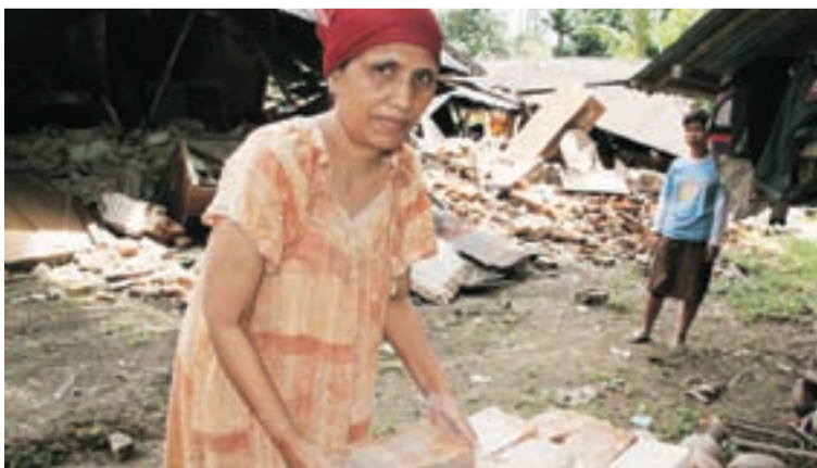
People who lost their homes in the Sumatra earthquake recycle bricks to rebuild.
