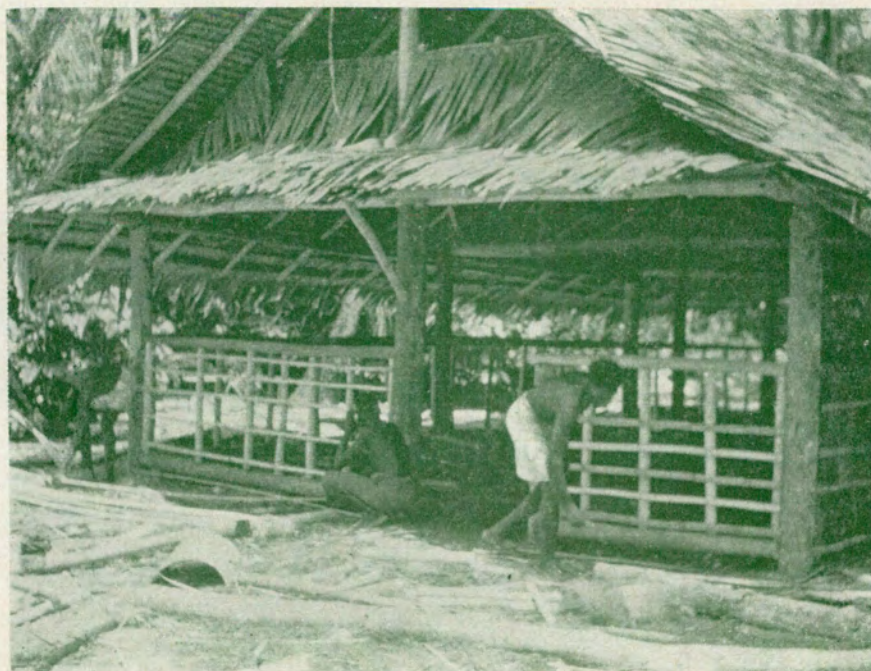
EXTENSION! Building new assembly room at Kihili Girls' School.
