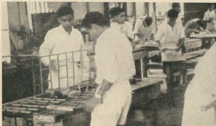
Below: THE TECHNICAL DEPARTMENT
