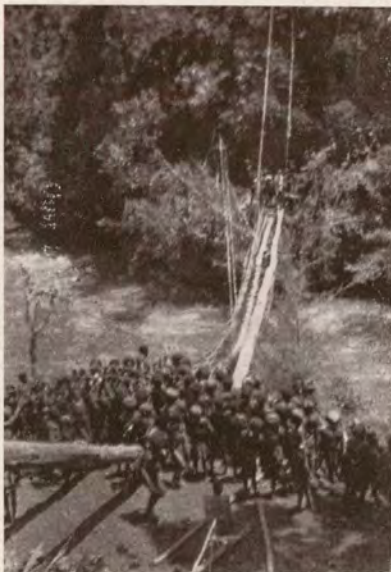
BUILDING THE MISSION BRIDGE AT MENDI
