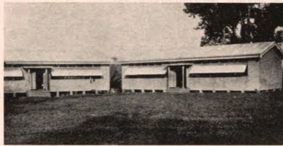
Dormitories at Navuso Agricultural School, Fiji—part of New Zealand Methodism's gift to Fiji after the hurricane of 1952.
