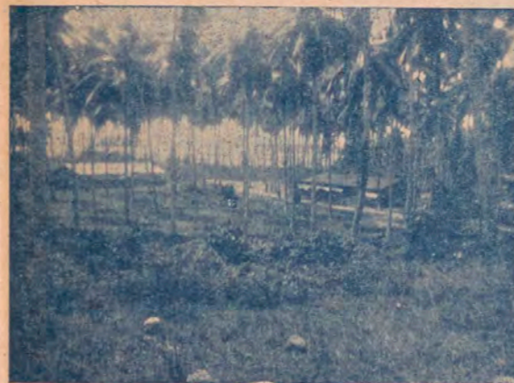
Bilua—showing temporary hospital buildings.
