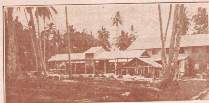
Mission Sawmill, Roviana, destroyed during the recent War. Steps are now being taken to erect a new sawmill at Koau, South Bougainville.
