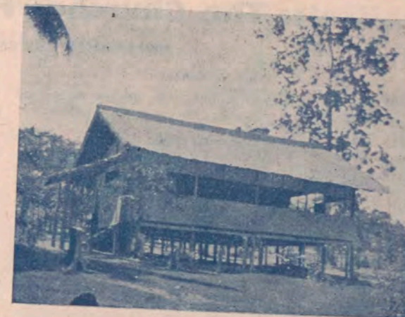
Simon Riqamu's house at Hoataraha—a masterpiece of native work.
