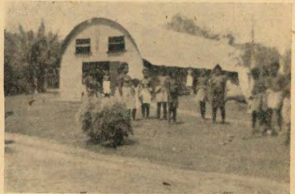
School Assembly Hall, Buin, 1948.
