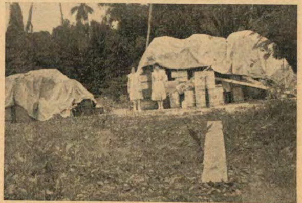
Goods stacked against the weather.
