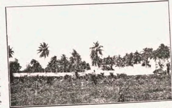
Long Bridge across Swamp at Kihili; badly damaged by the Earthquake.
