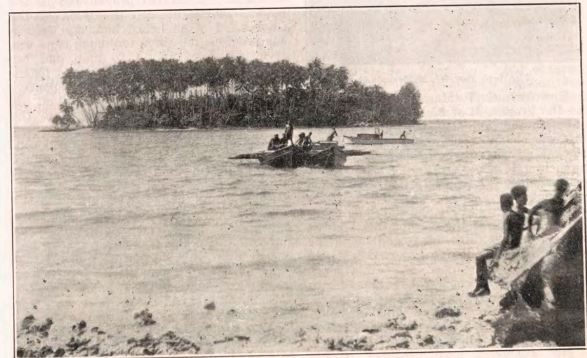
Landing building material for the Hospital at Bilua.
