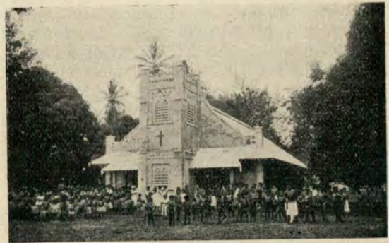
Bromilow Memorial Church, Dobu, Papua. Built in re-enforced concrete by native technical students under direction of Rev. M. K. Gilmour.
