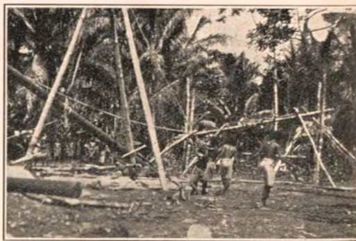
RAISING THE FIRST POST.
