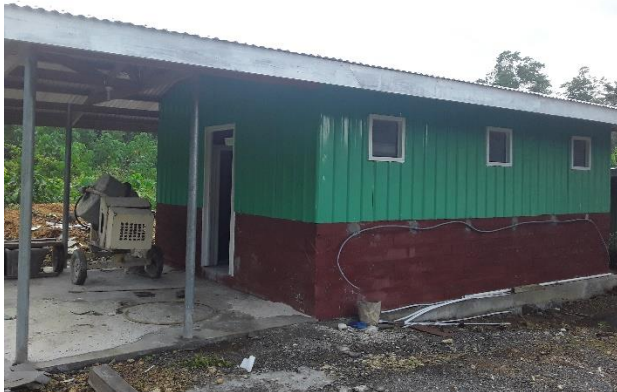
The Ablution Block for Girls is nearing completion
