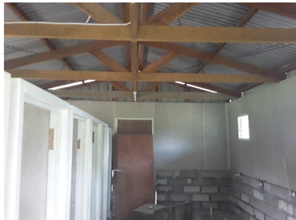
The interior view with construction work in progress
