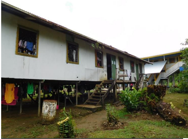
The old dormitory in the front and the new building behind it
