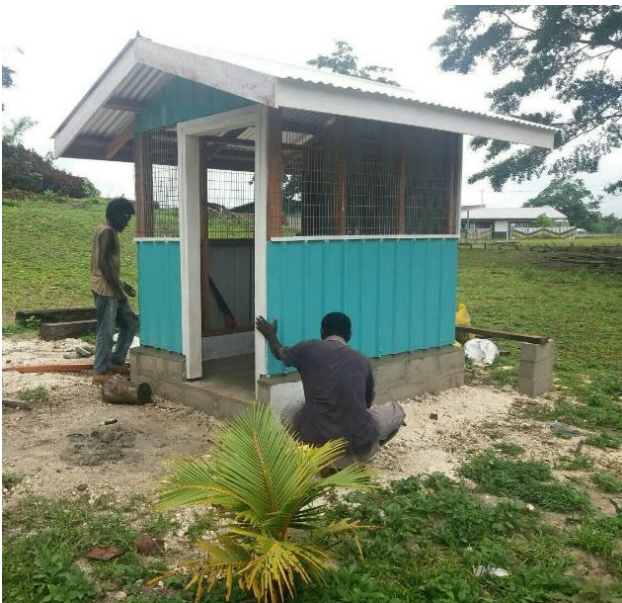
Pump House nearing completion
