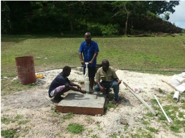
Work on the bore hole for water in progress
