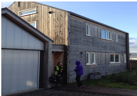
Zero energy house in Point Chevalier, Auckland.
